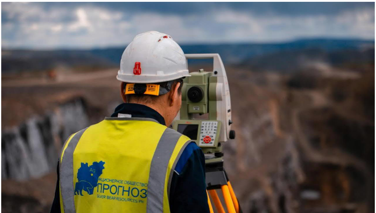
Mangazeisky Silver Project – Open Pit
