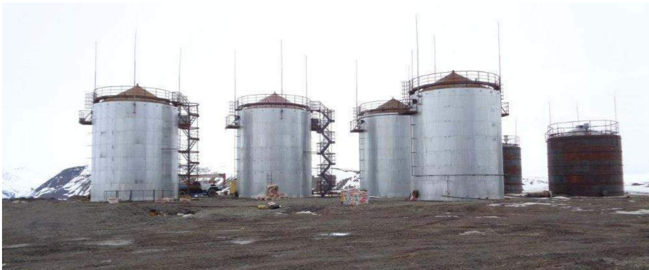
Fuel Storage Facility – Each with capacity of 1000 m 3
