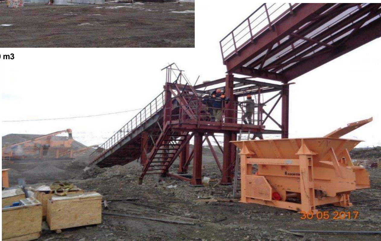
Installation of main conveyor belt and tension ladder
