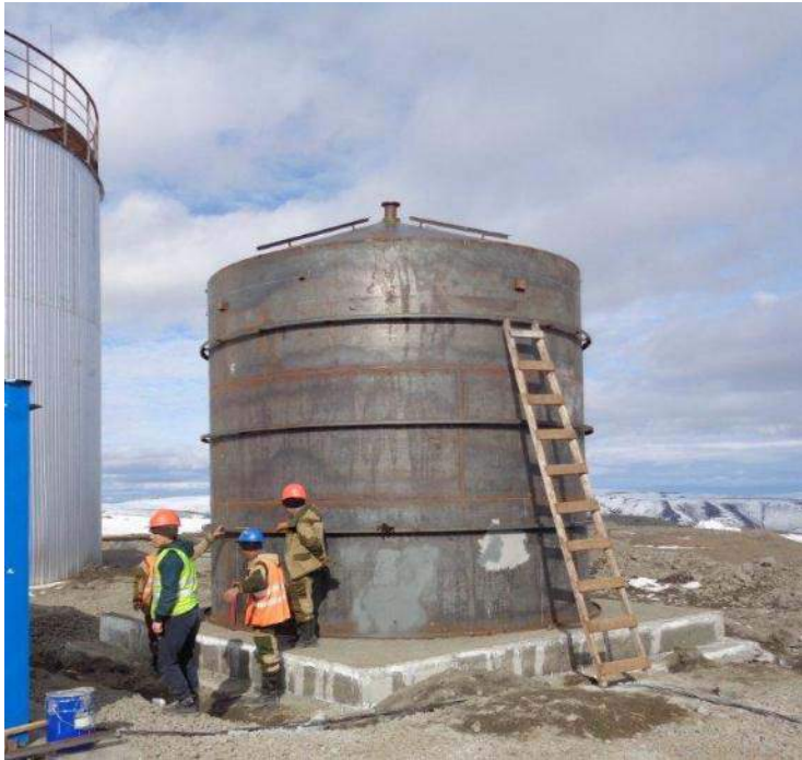
Installed 50 m3 drinking water tanks
