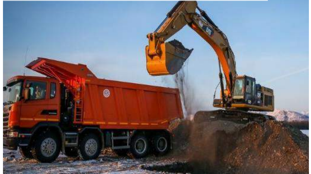
Silver Bear upgrades Local community infrastructure along ice road
