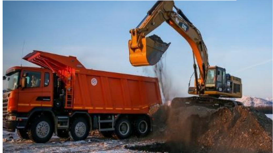
Silver Bear upgrades Local community infrastructure along ice road
