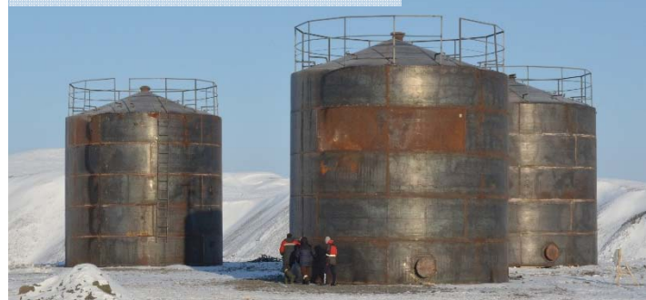
Fuel Storage Facility – Mar 2016
